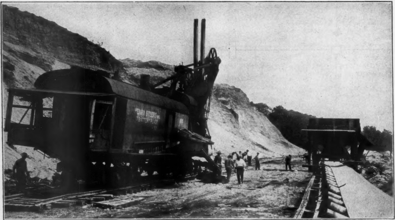
Large Shovel for Loading Pit Conveyor
